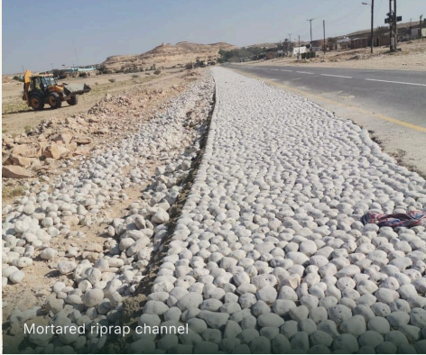
Mortared riprap channel Photographs are drawn from the company's protection works portfolio pages and are representative of the work type; they are not attributed to this specific contract unless captioned.
