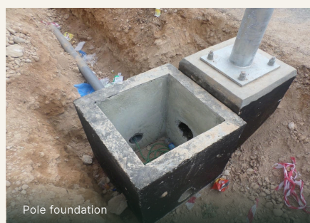
Feeder-pillar installation
