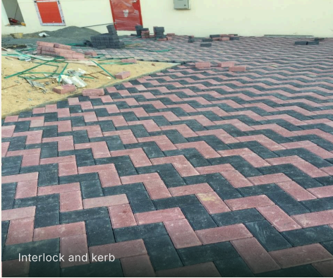
Interlock and kerb Photographs are drawn from the company's paving portfolio pages and are representative of the work type; they are not attributed to this specific contract unless captioned.
