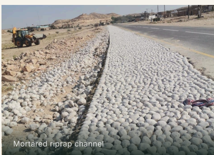
Line-ditch construction
